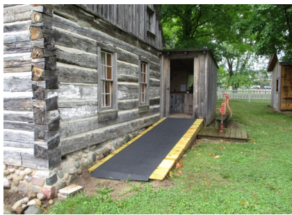
A ramp was installed at the Ott Family Cabin to make access easier to those with mobility problems. We would like to eventually install a sidewalk at our complex to connect all the buildings.
